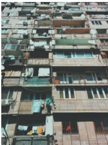
Logements, balcon- CC0 Domaine public
